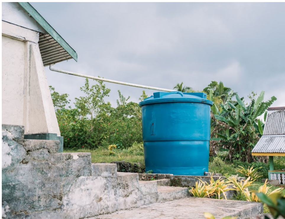
Caption: One of the 16 new water tanks that were installed across Parara, Kohigo Island, and Vonavona communities in Western Province's Ward 13.
