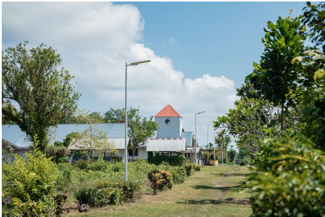
Caption: The 51 solar streetlights were installed along a 1.5km stretch in Madou, providing bright and reliable lighting for over 700 people for the first time.
